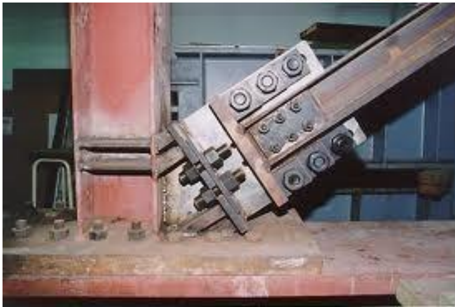
Bolted Connections
